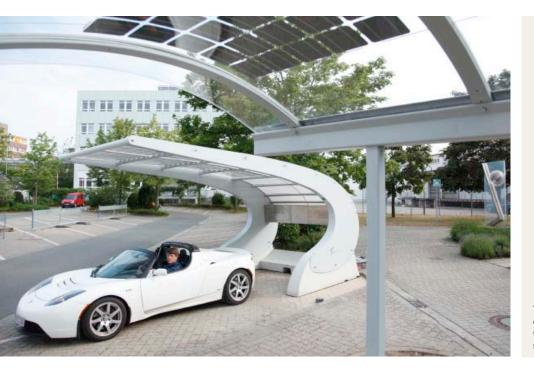
The SUNOVATION ECO TECHNICS carport combines design with functionality in an attractive way. Foreground a PLEXIGLAS® solar roof for the bicycle shelter.
