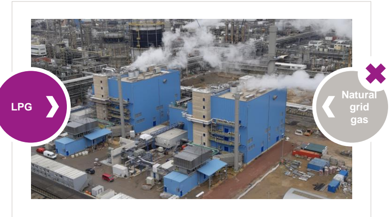
New gas power plant (Marl)
