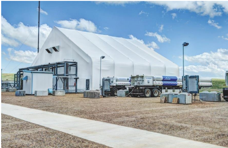
Photo caption: The picture shows the Linde engineered helium purification facility in Mankota, Canada, together with helium tube-trailers (right) for customer deliveries. (Source: The Linde Group).
