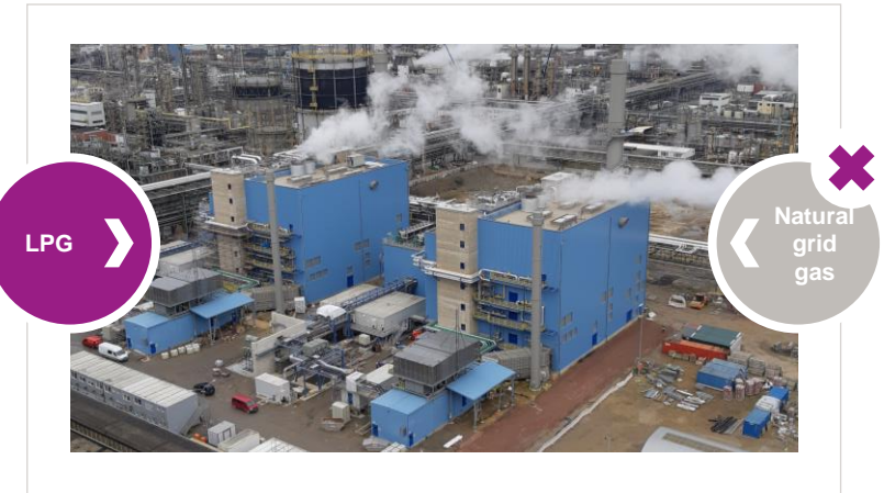
New gas power plant (Marl)
