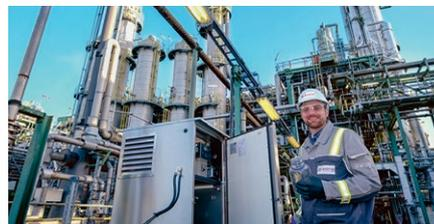
A new sampling station at the oxo plant in Marl (Germany) automatically takes daily samples of wastewater for analysis.
