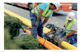
The polyamide 12 compounds of the VESTAMID<sup>®</sup> NRG series were specially developed for applications in the energy sector, e.g. for gas pipelines. They are characterized by high impact strength and stress crack resistance, which enable many years of safe service.
